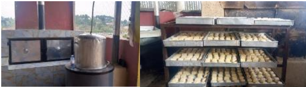
Left: First oven constructed and later demolished due to poor quality and capacity to burn enough bread;
