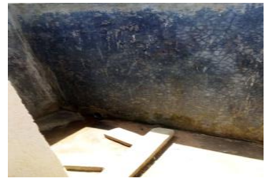
A door to be fixed on the washroom at Kirolo UMEA Primary School
