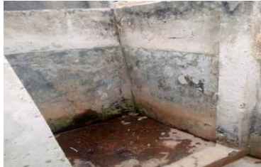
Washroom to be repaired and fix door at Maganjo UMEA
