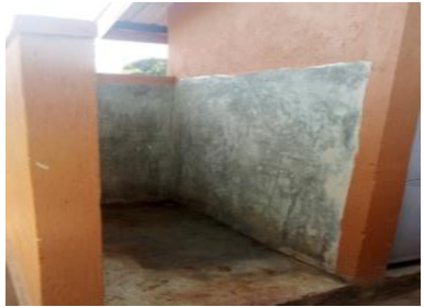
Fitting a door and roof at Ssanga C/U Primary School
