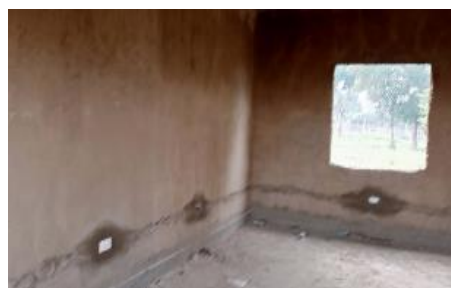
It will be fitted with windows and a door soon to commence operations.
