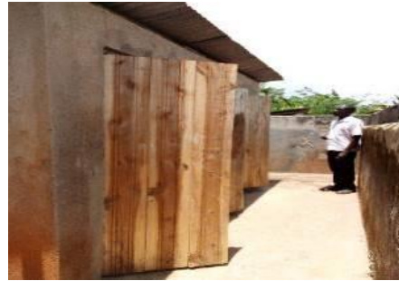
<After> Toilets with fixed doors
