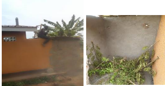
<After> The school constructed a changing room which is still not ready for use as the floor is still wet
