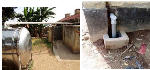
<After> Gutter and soak pit renovated
