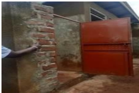
<After> Washroom door fixed with a lock. Pending is plastering.
