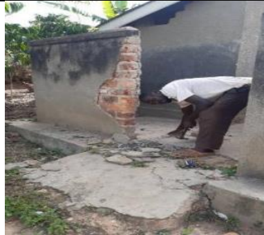
<After> Girls' washroom's dirty floor being improved
