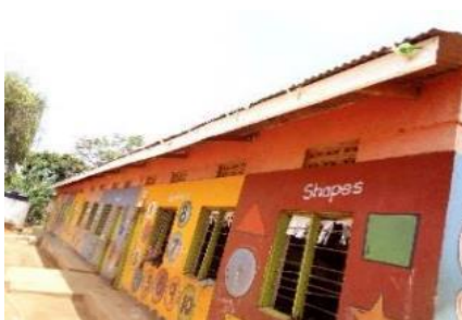
<After> Gutters holders have been fixed and gutters will be fixed
