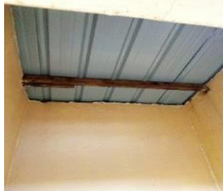
<After> New iron sheets were fixed
