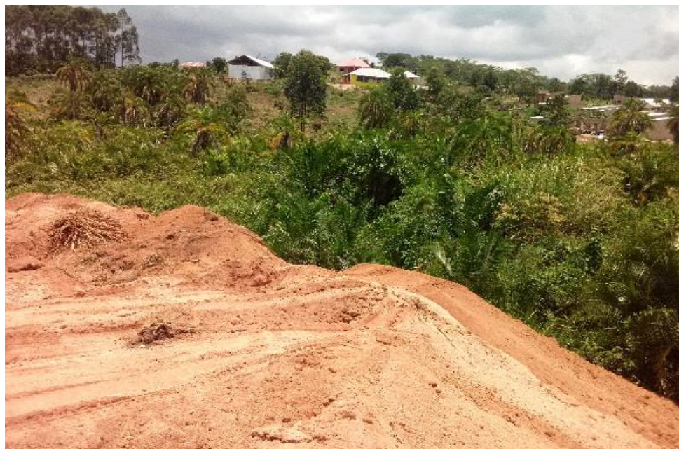
Wetland land filling in Lusalira village –Kibalinga sub-county.
