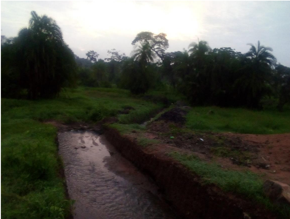
Drainage channel constructed to reclaim land from a wetland, in Kiyita village Nabingoola sub-county
