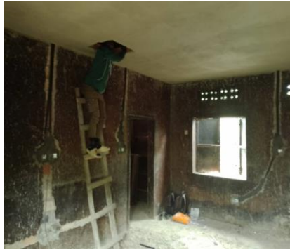
During maintenance of the inside part of the radio house
