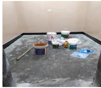
After painting of the inside part of the radio house
