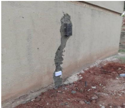
During maintenance of the outside part of the radio house
