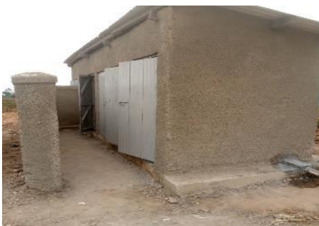
Toilets with fixed doors
