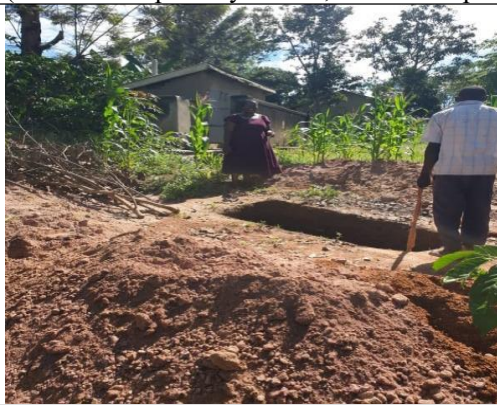
Construction pit latrine of Kitagobwa primary school
